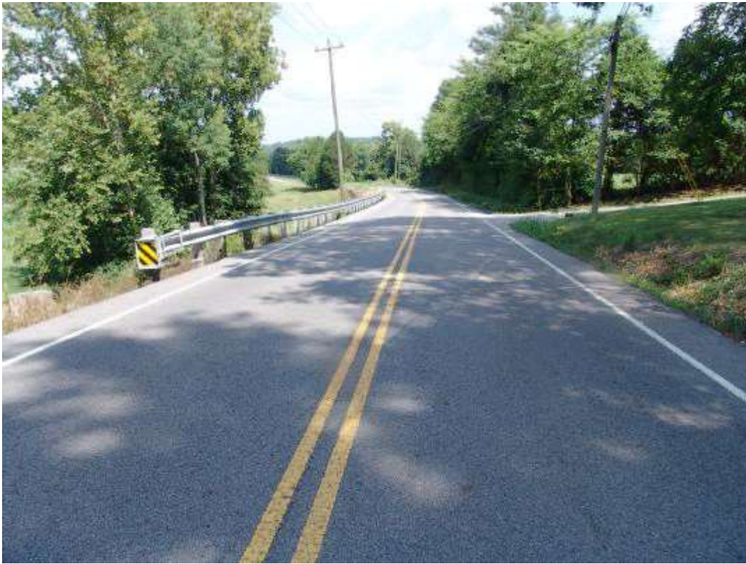
Photograph 0011: Northbound Canyon Road. Guard rail extended approximately 105 feet south after collision.
