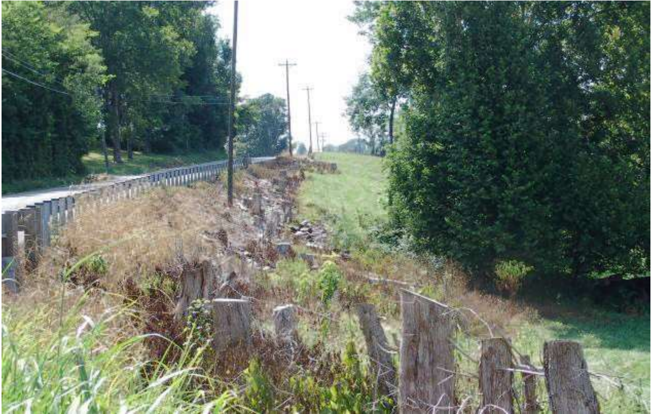
Photograph 0015: View of the new section of guard rail and the slope of terrain away from the roadway.
