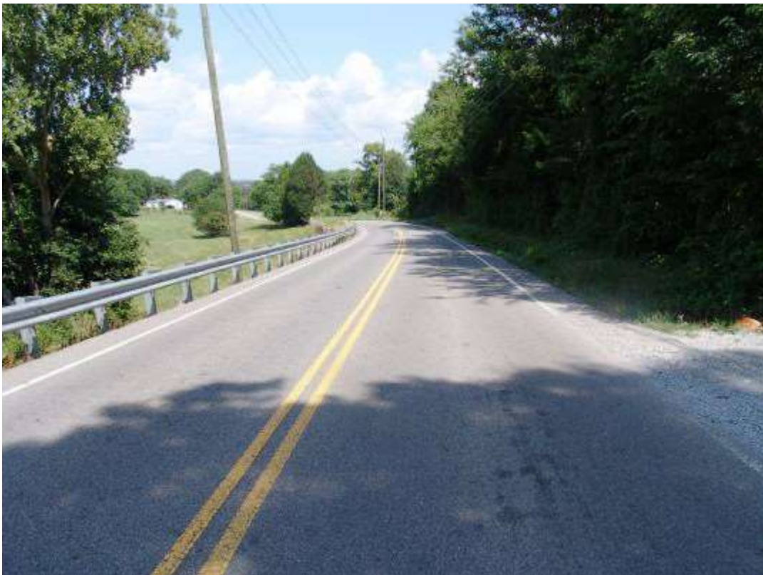
Photograph 0012: Northbound Canyon Road. Utility pole remains on the left side of the roadway. New section of guard rail is on the left side of the roadway. No tire marks are visible on the roadway.
